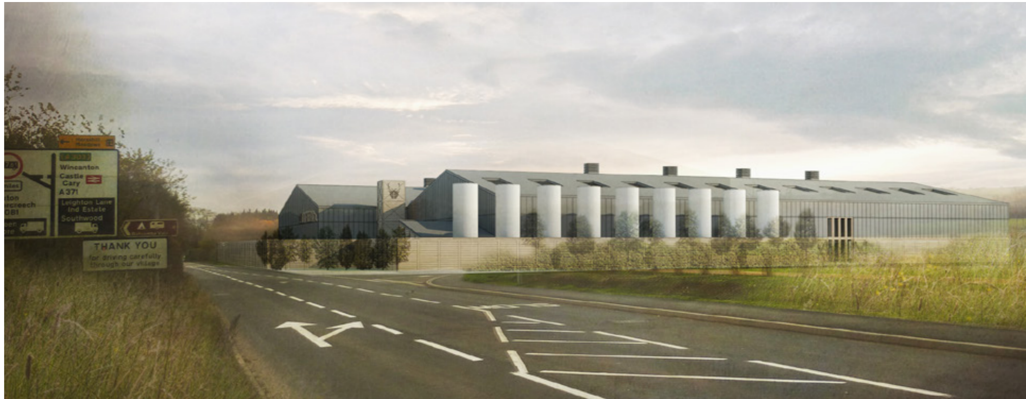
View of site from Prestleigh to the north-east
